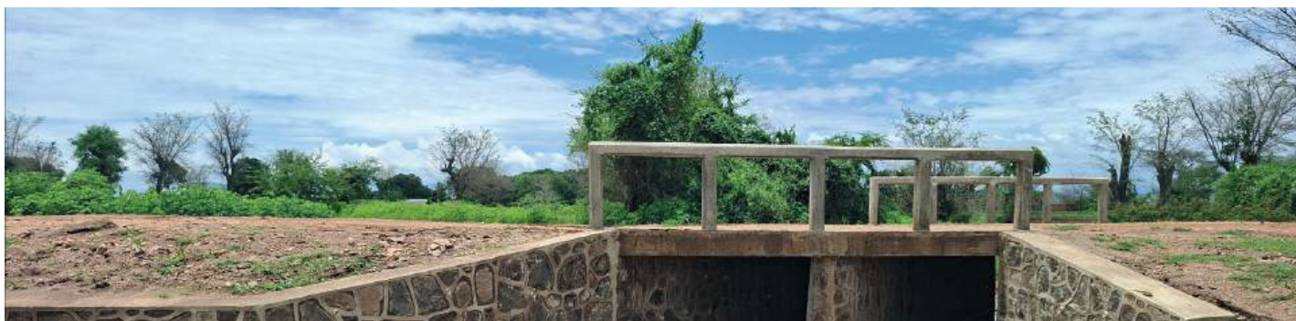
Completed Kambwe-Silu Road Box Culvert. Picture by George Mponda.
