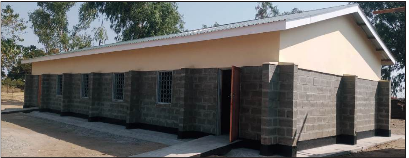
New block at Kakwale Primary School. Picture by Wanangwa Tembo.
