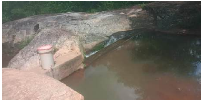
Intake weir at Mfundazi Water Supply Scheme.
