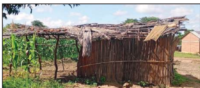
A structure which was used as a classroom due to the shortage of classrooms at Kadagwantipenya.
